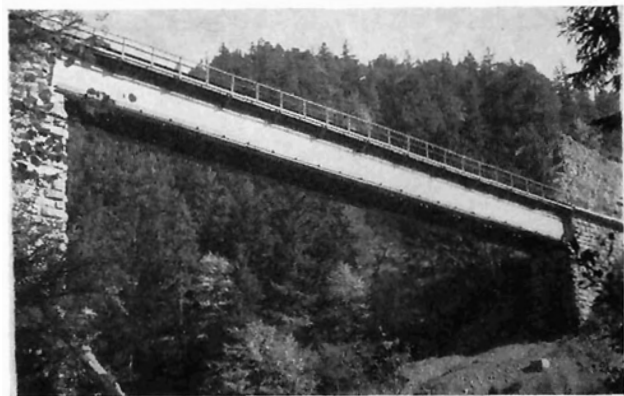
Fig. 7a: Disassembly of the old bridge
