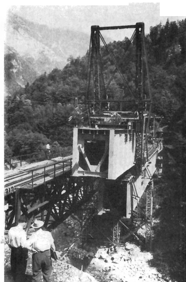
Fig. 4c: New bridge, erection
