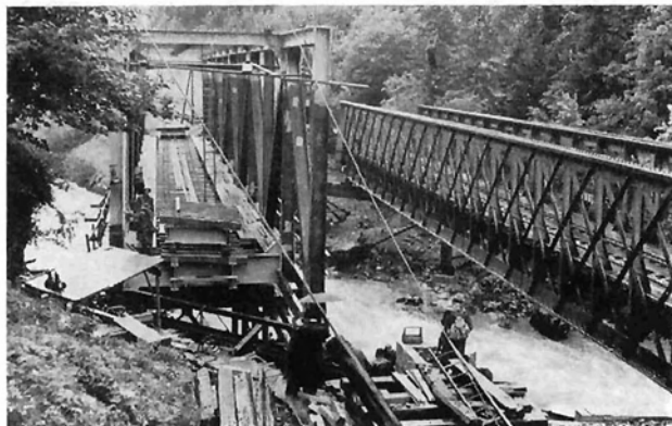
Fig. 8: Kummer-Bridge; Erection
